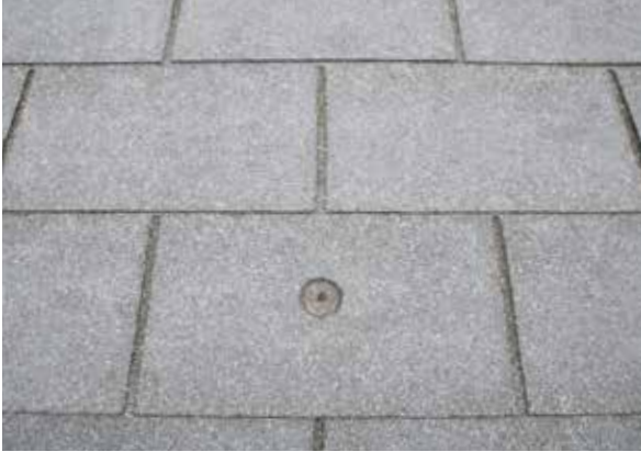
THREE TAB shingle roof
